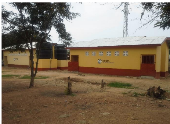
Two of the toilet facilities constructed at the Gbawe cluster of schools in Ga South in the Greater Accra Region
