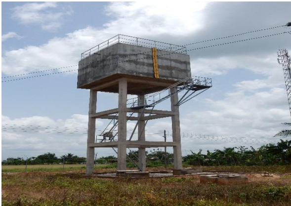
The high level tank in Acherensua
